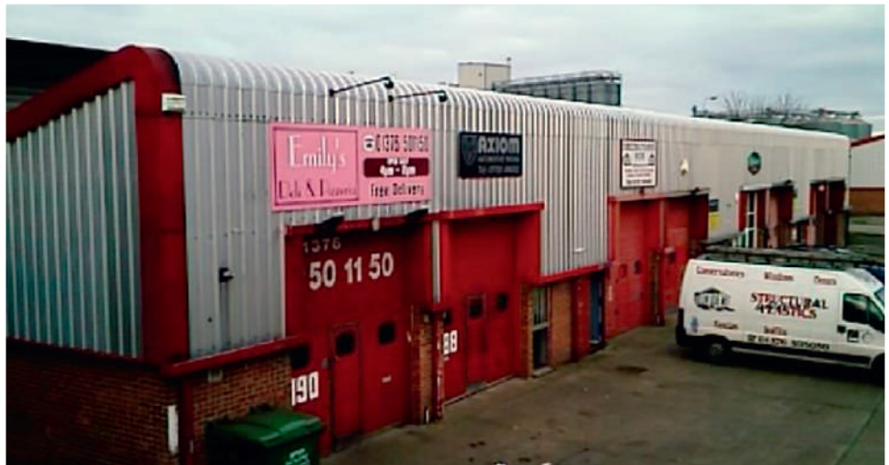
Figure 1.26 Small specialist companies are often located in units similar to those shown here
